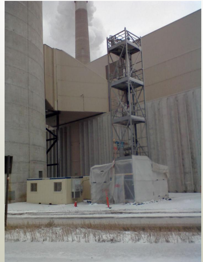
Xcel's Sherco Station
