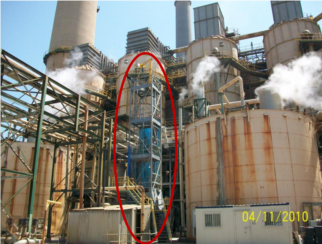
Luminant's Martin Lake Power Plant
