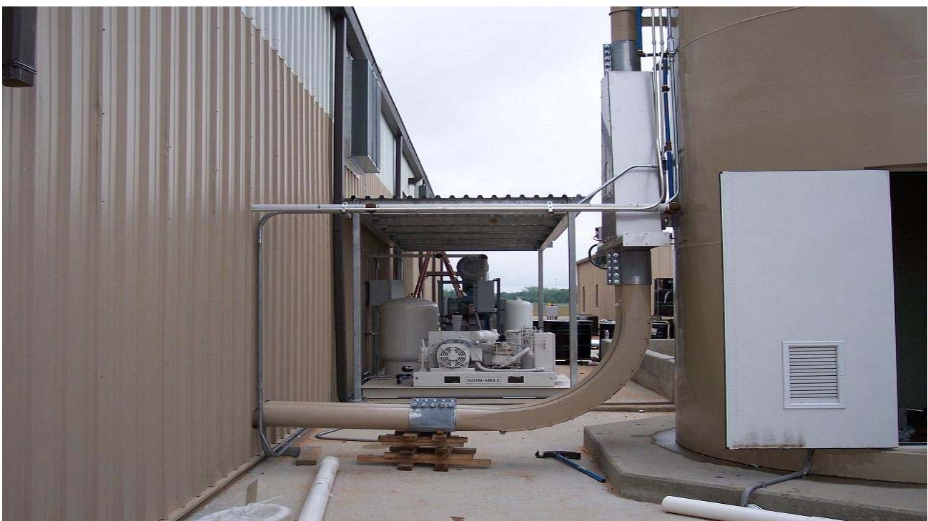
May 15, 2009 – Mechanical and process equipment installation continues.
