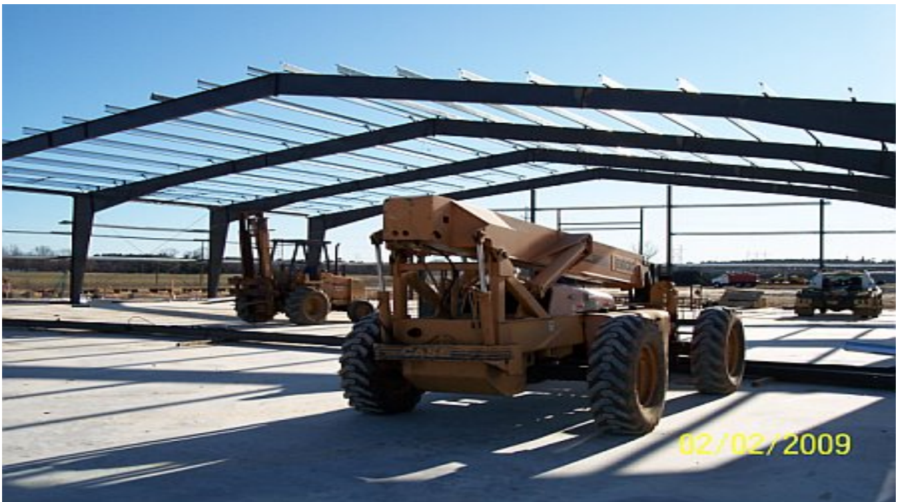
February 2, 2009 - Warehouse steel erection.
