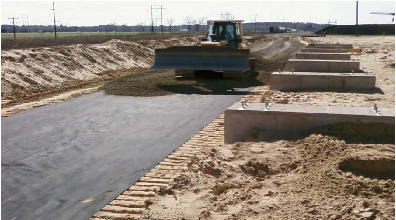
February 6, 2009 - Rail spur sub-grade
