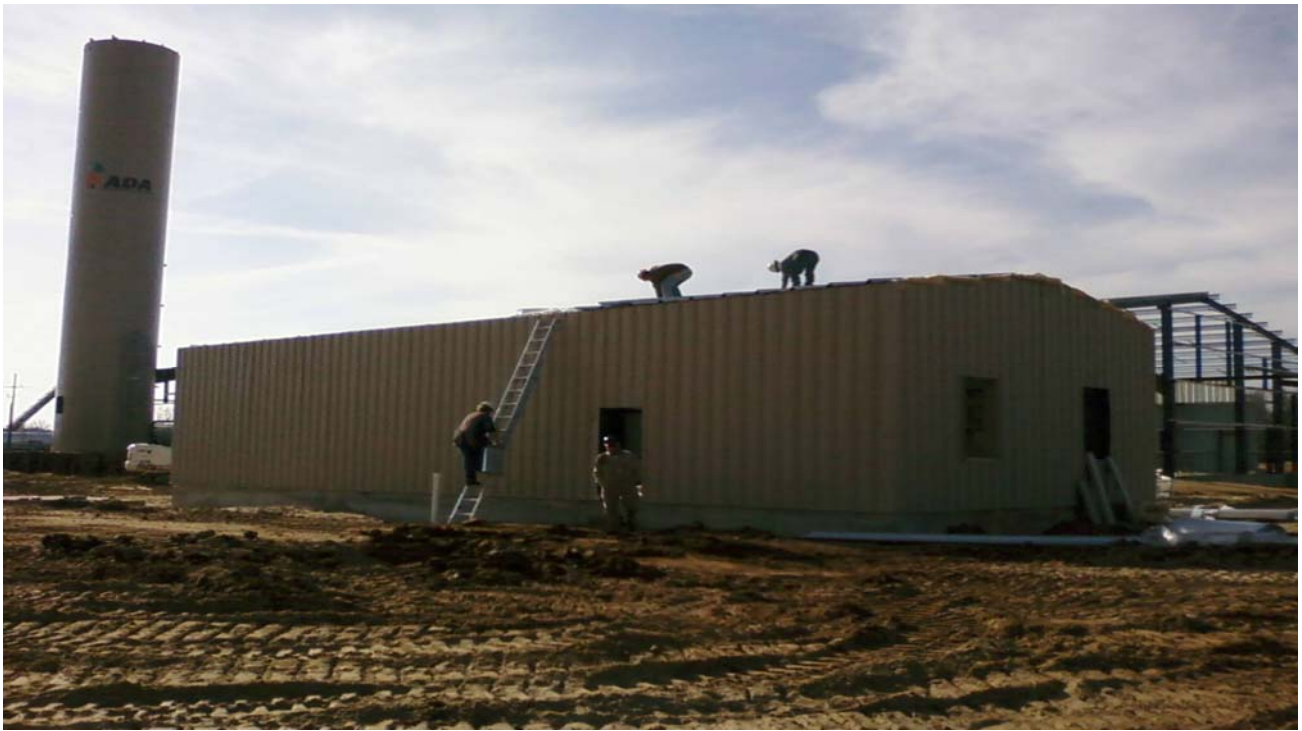
January 5, 2009 - MCC / Control Room building
