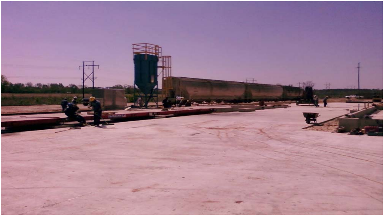
April 17, 2009 – Load out area continues to take shape.
