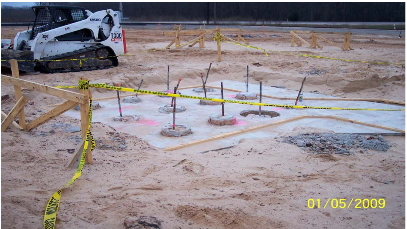
January 5, 2009 - Piles for mill foundation
