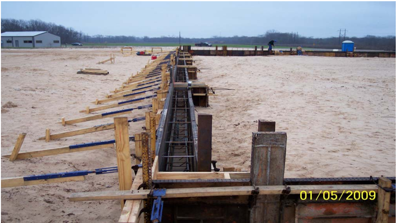
January 5, 2009 - Grade beam forms for warehouse foundation.
