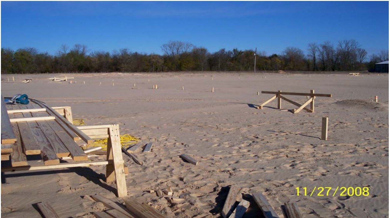
November 27, 2008 - Beginning to lay out site
