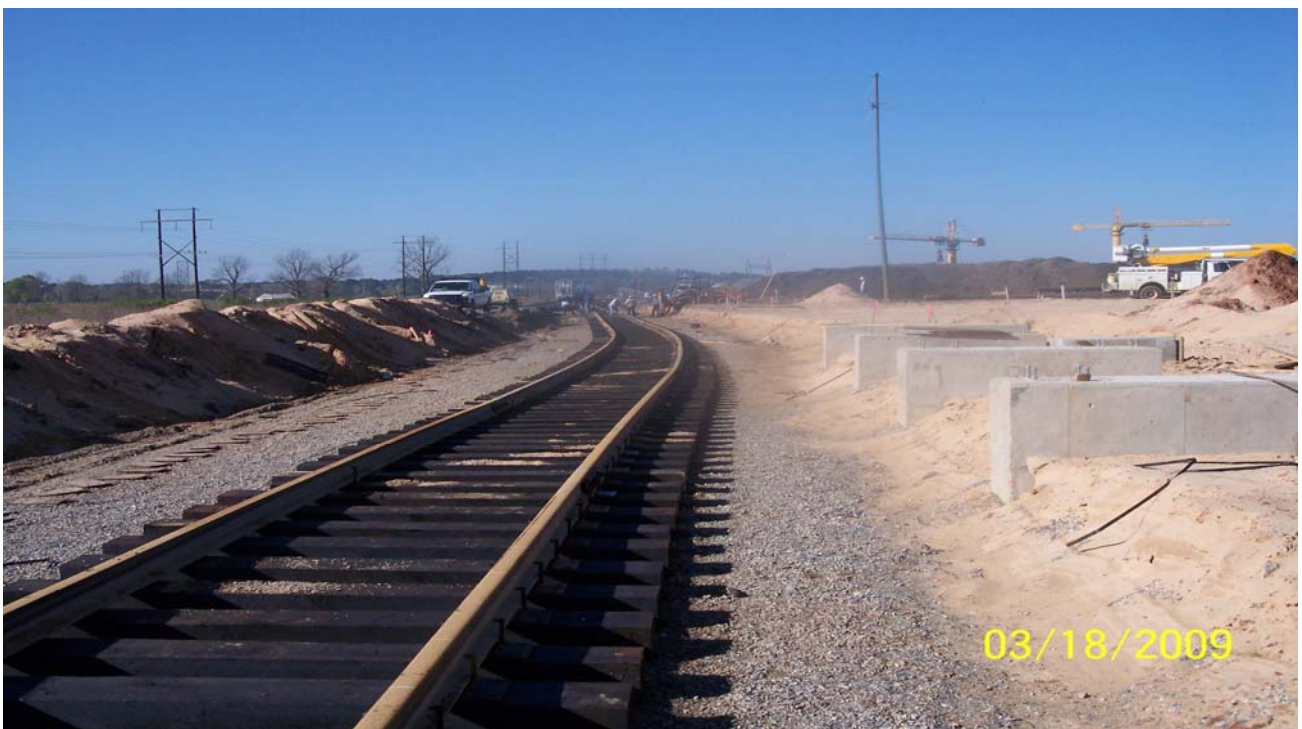
March 18, 2009 – The rail spur nears completion.
