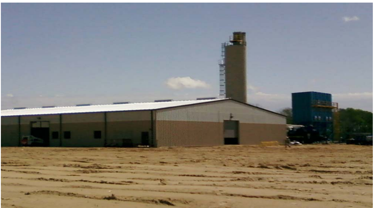
April 17, 2009 – Warehouse nears final acceptance.
