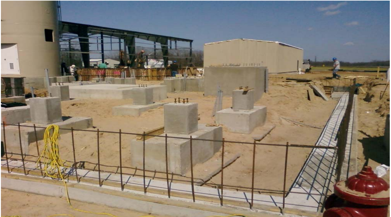
January 5, 2009 - Equipment foundations and process area containment wall going up.
