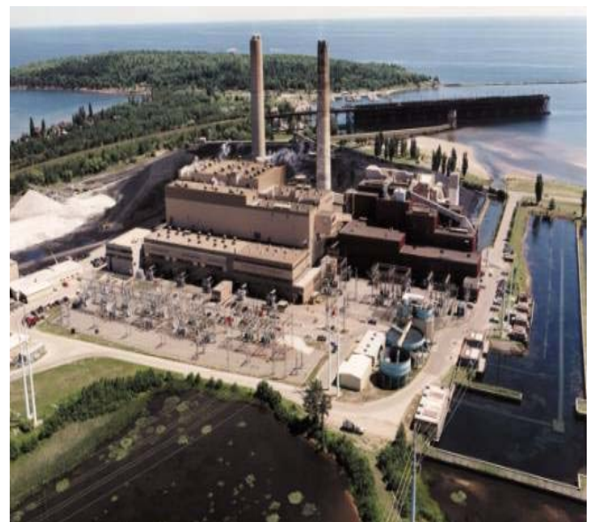
We Energies—Presque Isle Plant
