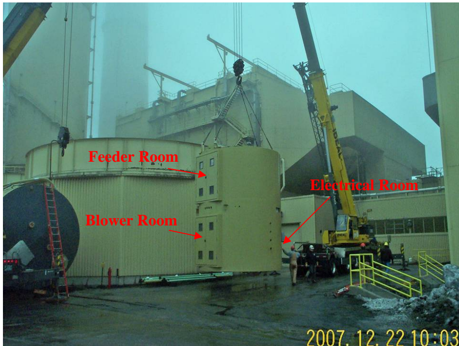
Figure 2. Installation of PEM.
